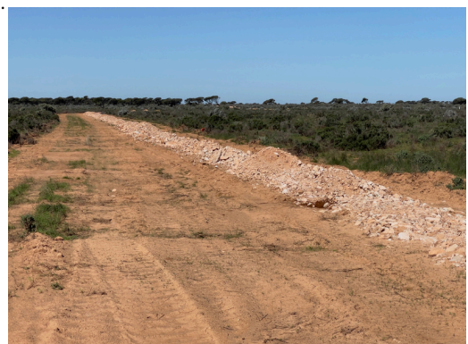
Telstra Trench, Old Eyre Hwy, south of Koonalda Homestead. Photo by Clare Buswell.
