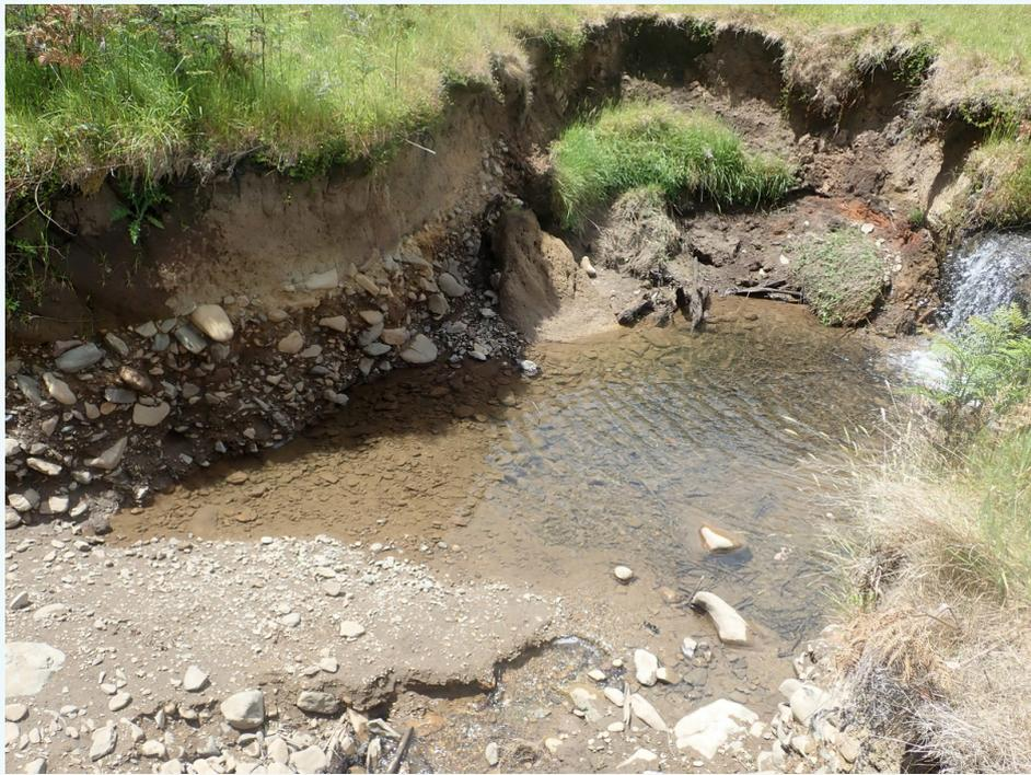
Figure 5: Erosion of the surface channel undermining fencing
