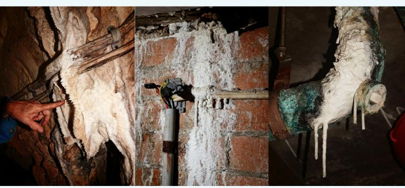
Fig 4. Calcite over the power cables in Hill Cave, Abercrombie, NSW
