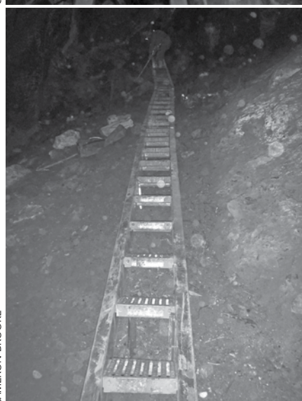
Before (upper) and after (lower) repair of the aluminium walkway in the lower entrance of Kubla Khan Cave
