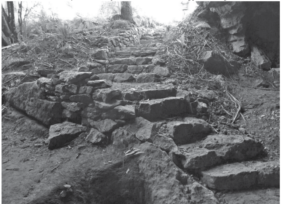
Detail of integration of existing bank rock structure for viewpoint landing
