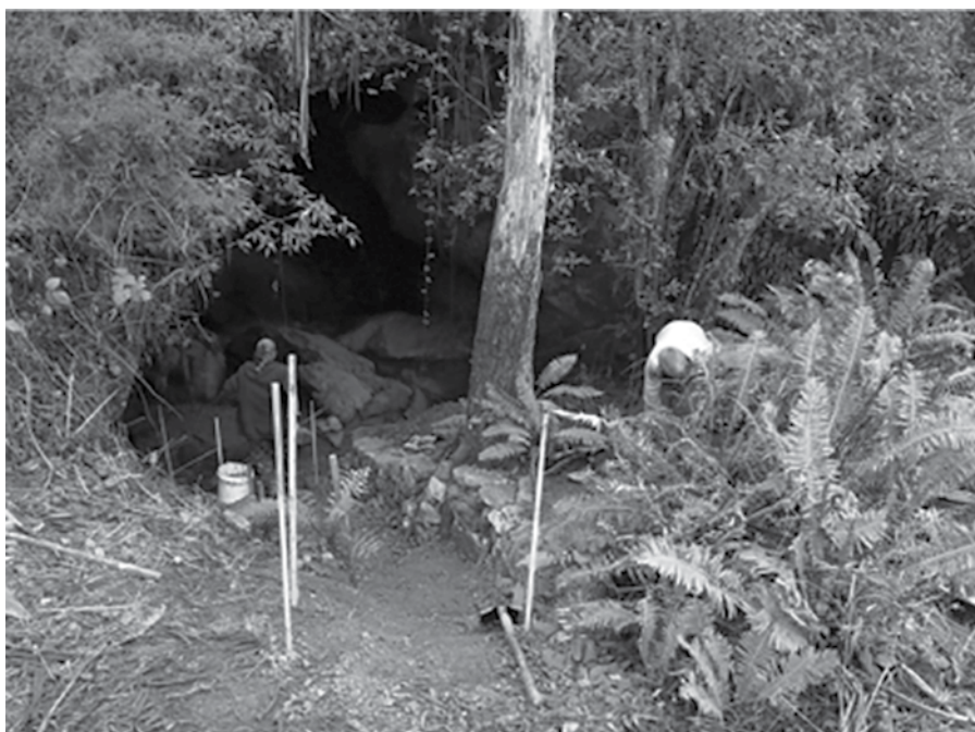
Material from excavating the steps' foundations backfilled around the tree's exposed roots
