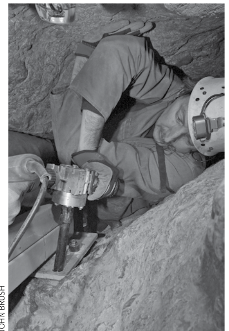
Drilling the anchor holes.
