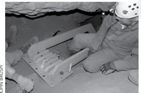
Levelling the bridge frame.
