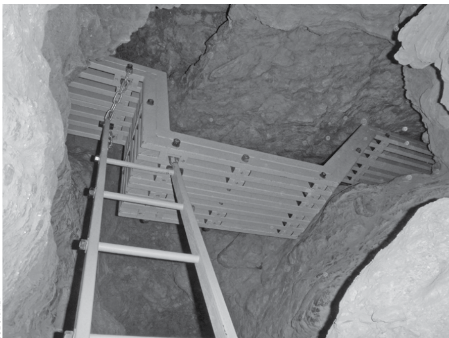
The bridge and ladder installed over B4 Kings Cross void.
