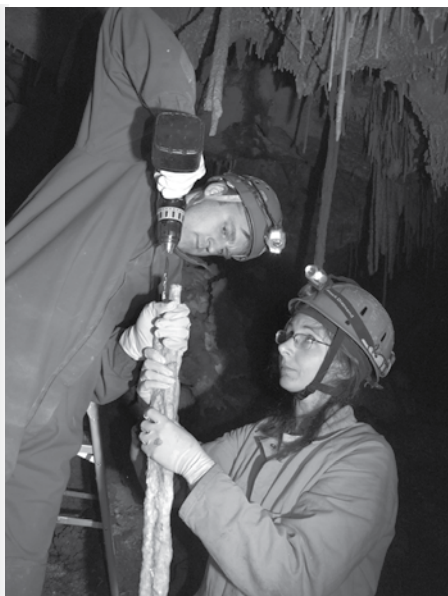
Enlarging the pin hole before final connection to the roof
