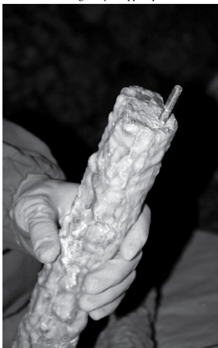
Threaded pin glued in a more solid section
