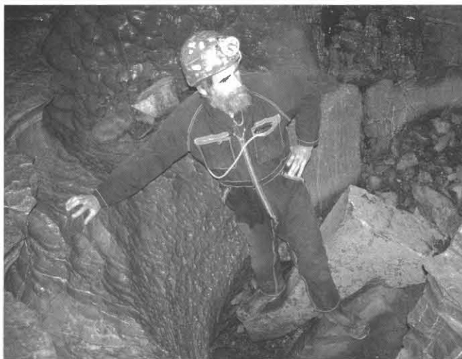
Tom Porritt standing on top of new rock fill dam in Cephalopod Creek.
