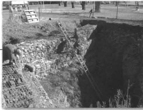
All Gabions now filled and in place.
