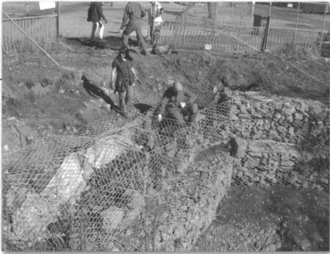
Top row of wire Gabions in position.
